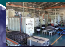
Vacuum heat treatment facility in Incubation plant
