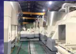
New heat treatment facility in main plant
